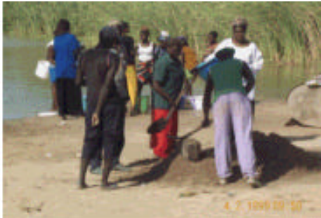
Civil works near the river
